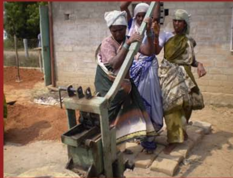
Our workers at the mud block production site.
